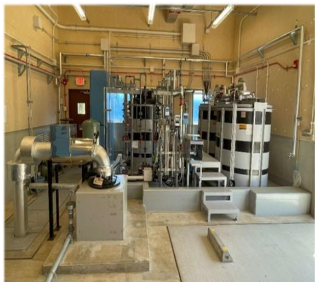
Figure 2: Sodium Hypochlorite & Fluoride
