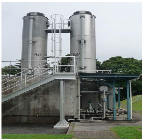
Figure 1: Air Stripper Tanks
